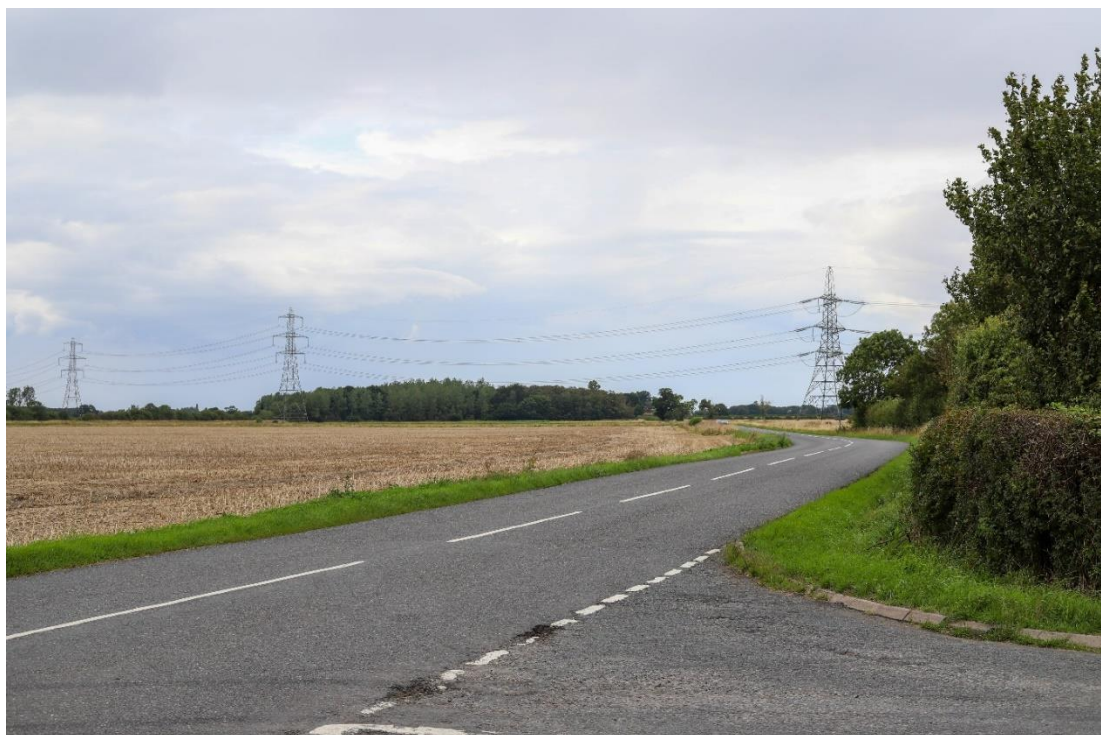
Plate 2-5: 400kV overhead powerlines carried by pylons within surrounding landscape
