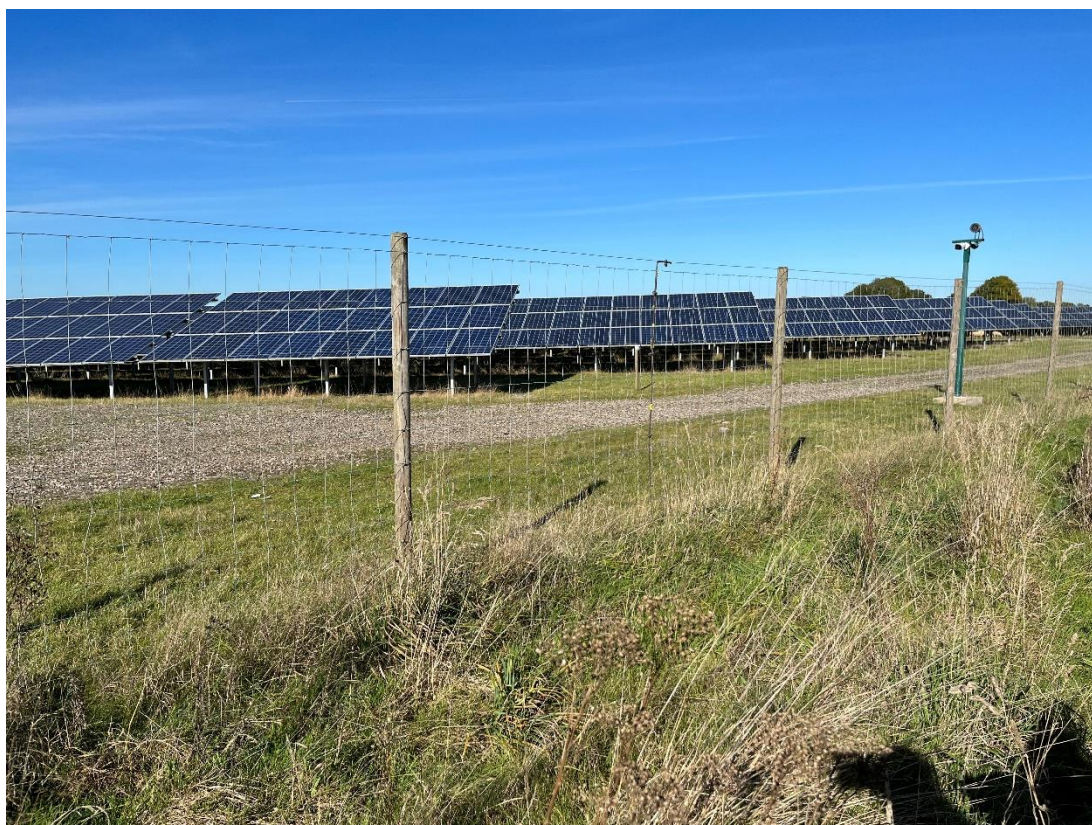
Plate 3-9: Example of mesh stockproof fencing and a metal perimeter CCTV pole
