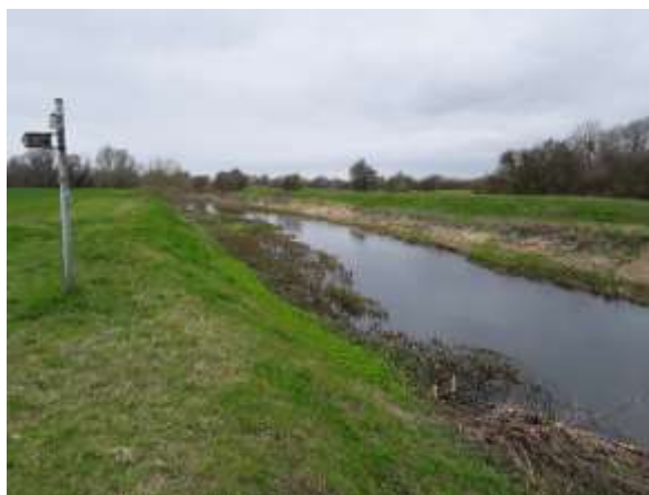
Photo 8 – River Witham at TN21
