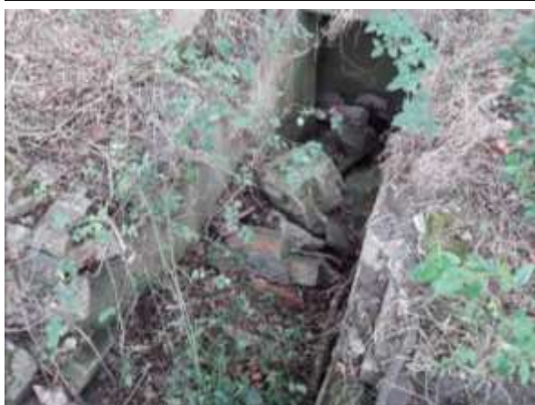
Photo 17 – Underground structure at TN36
